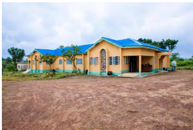
Renovated Border Post Building, Sierra Leone
