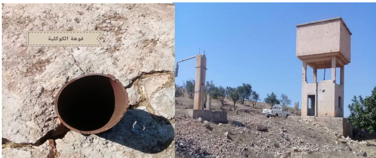
Figure7: Kokliah groundwater well
