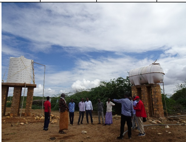
Kerinbile kebele constructed elevated roto tank with 10m 3 tank
