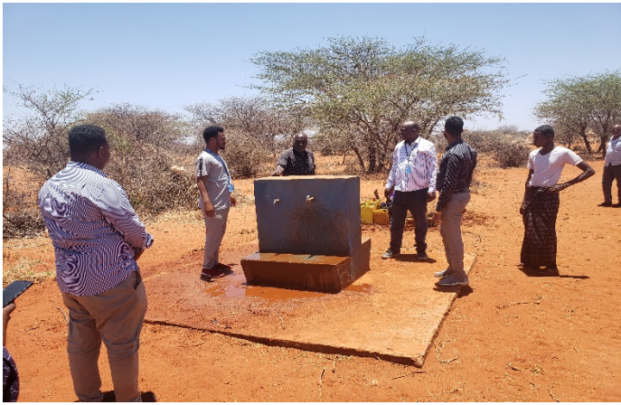
Nagardale Borehole rehabilitation through construction of Elevated masonry roto-stand and waterpoint
