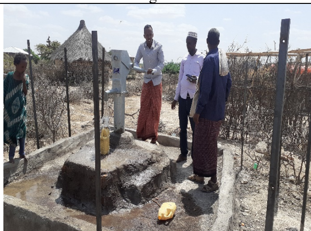
Dalada kebele rehabilitated hand dug well
