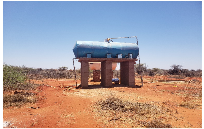
Nagardale Borehole rehabilitation through construction of Elevated masonry roto-stand and waterpoint
