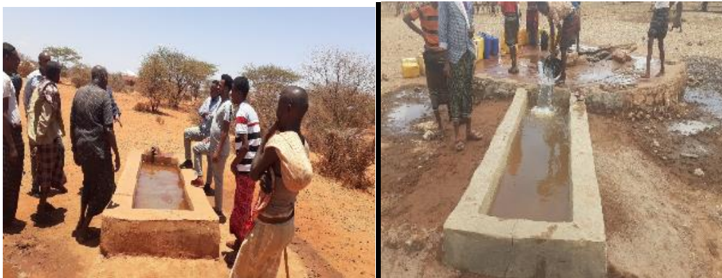
Cattle troughs constructed in Warder Woreda
