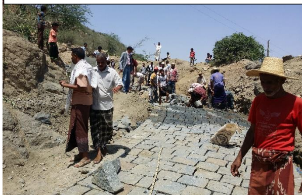
Access road building for IDPs and Host communities
