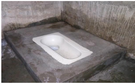
Low-cost Latrine through the provision of sanitation kits -
