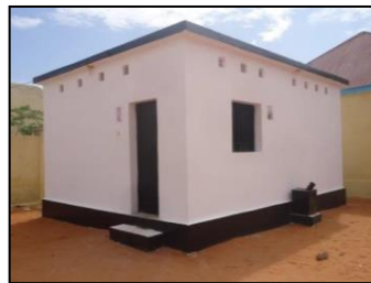
Munitons storage after refurbishment
