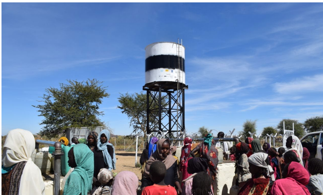
A newly renovated water yard in Wannu village, Sirba locality West Darfur. The Water yards which are located close to communities ensure the safety of girls who do not have to walk long distances to fetch water. (Photo credit: RCDO, West Darfur 2022).
