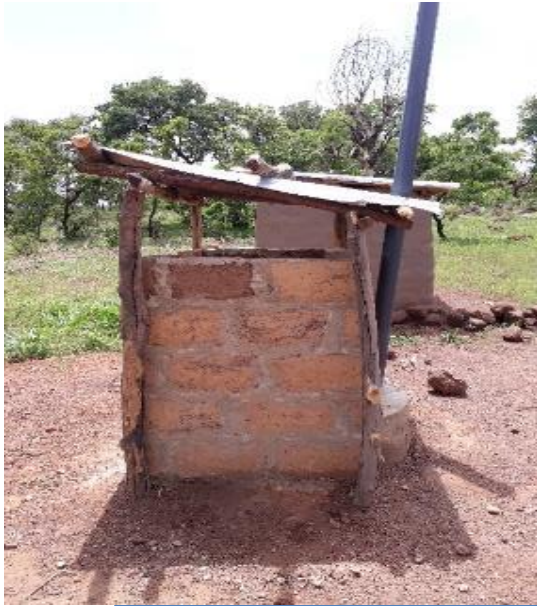
Photo 6- A flood resilient household toilet structure to poor households (showing installed)
