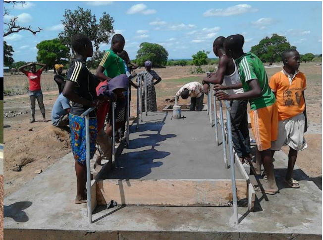
Photo 2 – Construction of an elevated platform
