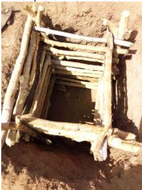
Photo 3 - Local lining option using timber built by CTV
