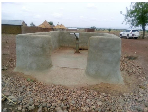
Photo 12 - Improvement of water sites, Atuba Mognori
