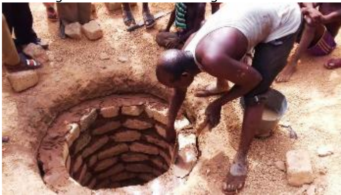
Photo 5 - Local lining option using bricks built by CTV
