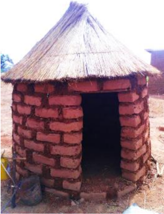
Photo 4 - Completed household toilet built by a community technical volunteer
